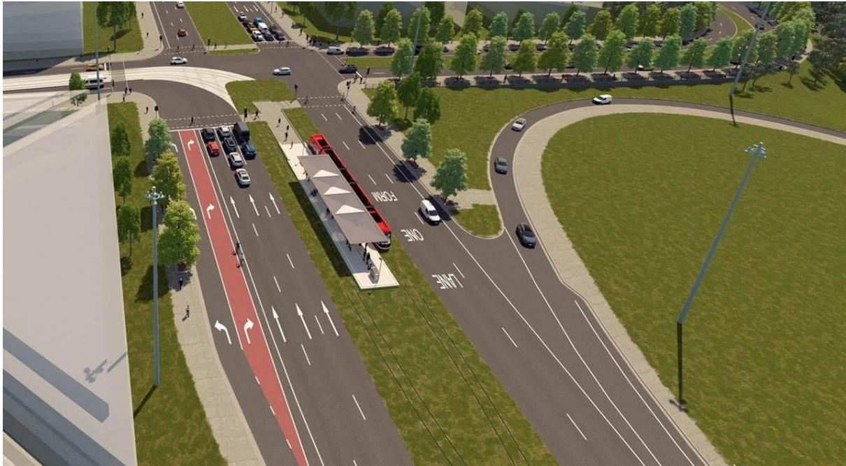
**Figure 2:** Bus priority turning lane on Commonwealth Avenue
